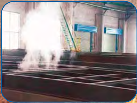
Curing of cement
